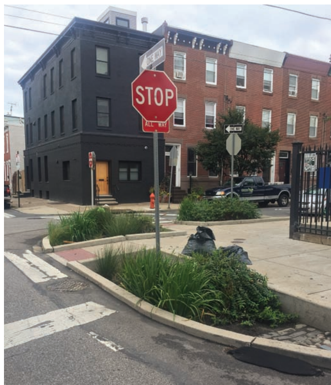
A stormwater utility not only supports activities that improve existing infrastructure and reduce flooding but also works to support new construction, including green stormwater infrastructure like this “green street” in Philadelphia.
