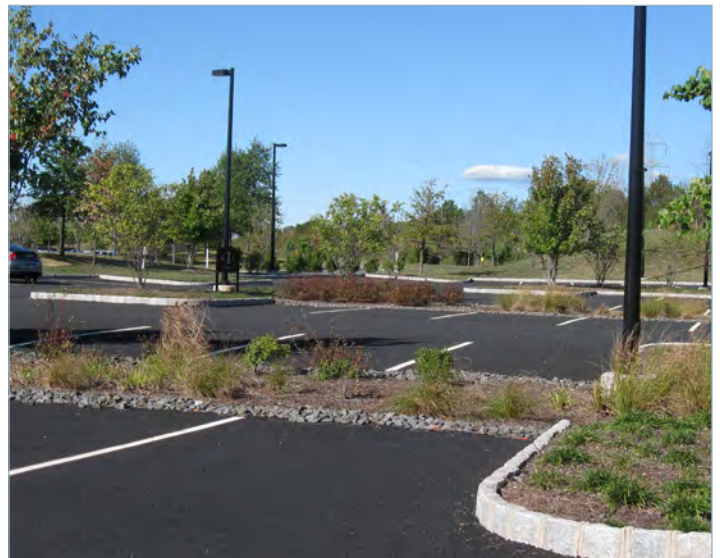
Parking lots, notorious for generating stormwater, can be "greened" with the addition of pervious pavement and vegetated swales, such as in this example from the New Jersey Department of Environmental Protection.
